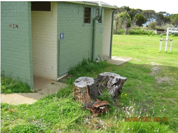
Toilets – Remove trip / fall hazards in adjacent area and pathways, repair broken windows, identify and resolve the source of flooding on the floor, ensure external lighting is available to illuminate the pathway from the hall at night. Should the toilets be developed to include a disability toilet, ensure pathways have the correct width and fall.
