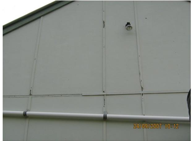
Exterior – Repair or replace broken battens.
