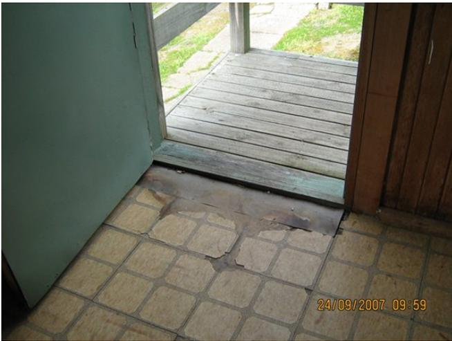
Flooring - Repair or replace vinyl floor covering, and install weather strip to door to prevent storm water from running under the door.
