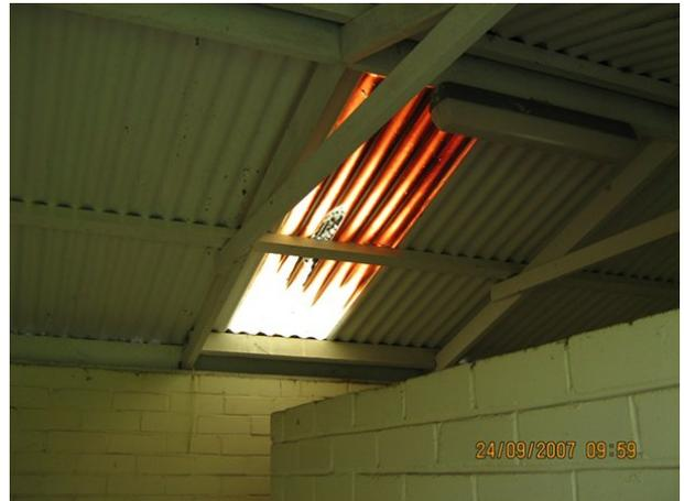
Skylight in toilets – Replace broken sheeting And install wire mesh under the sheeting to prevent a person falling through.
