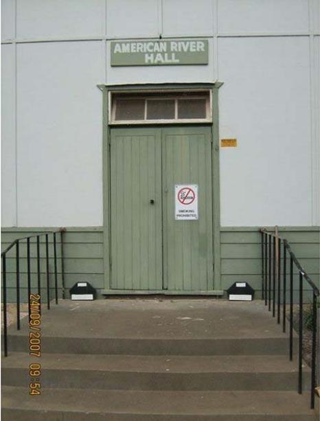
Front entrance – Ensure doors are structurally sound and weather proof. Replace door handle to comply with Emergency Exit door handles.
