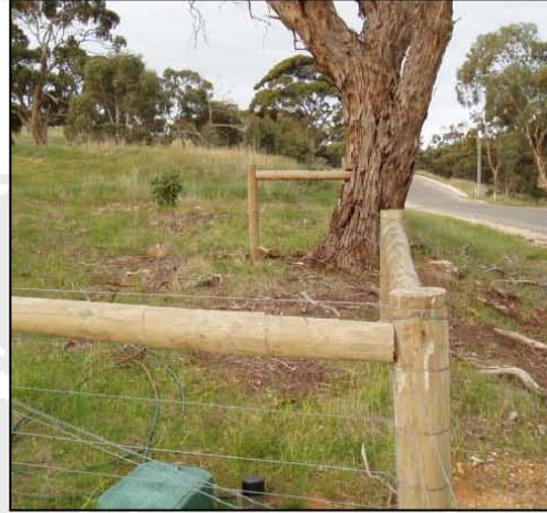
Photographs showing a simple strut arrangement that allows a fence to deviate for a short distance around a tree. Wires are not attached to the tree minimising potential damage to the tree.
